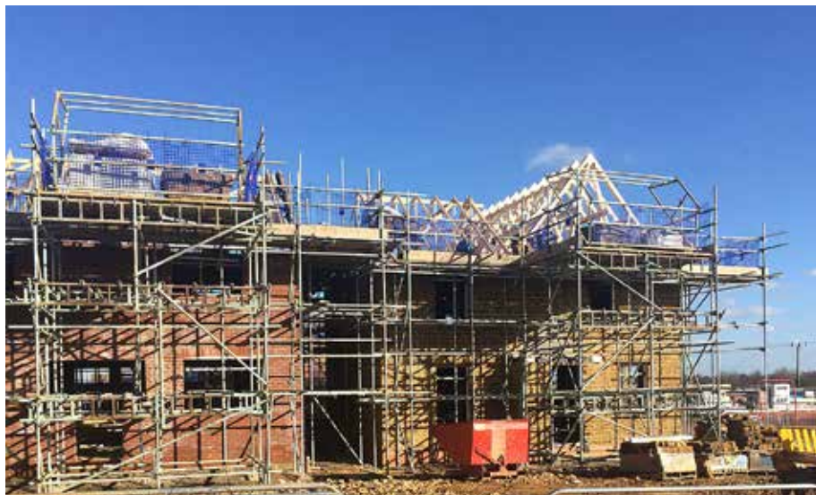
The first houses on the new estate are due to be finished this summer. Work will continue until 2017.
