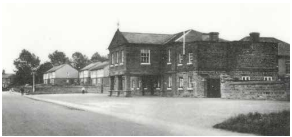
People used to fear being sent to the Brixworth workhouse on Spratton Road, which at one point housed 2,281 people.
